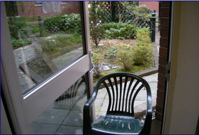
A & E staff room/kitchen door propped open
