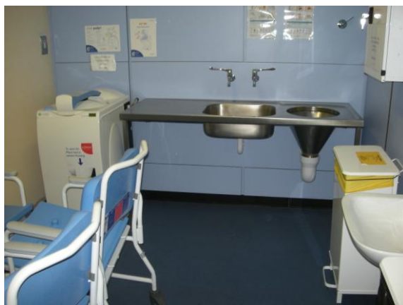
Picture 3: Refurbished dirty utility area
