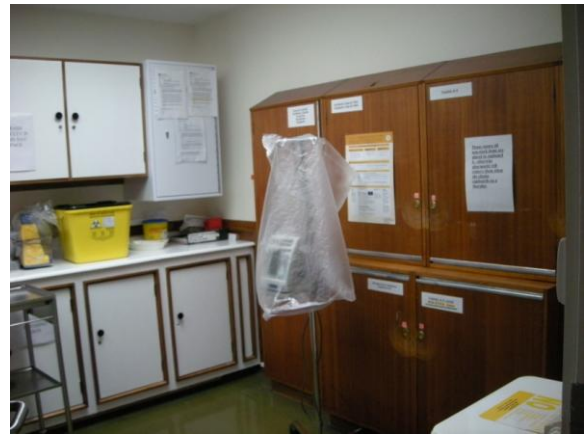
Picture 3 Tidy treatment room, worn wooden cupboards
