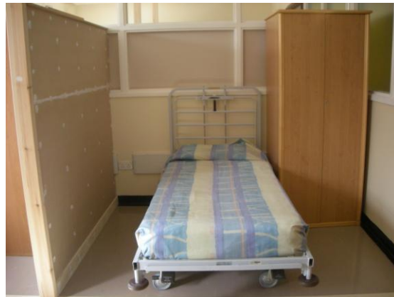
Picture 3: Bed area under construction
