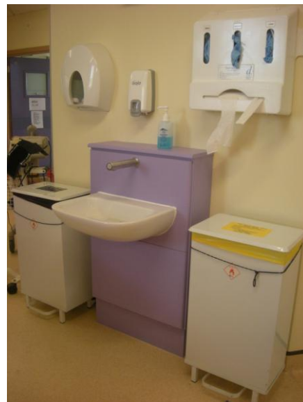
Picture 5 Typical clinical hand wash sink
