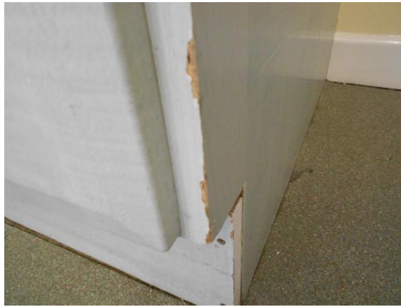
Picture 2 Damaged cupboard
