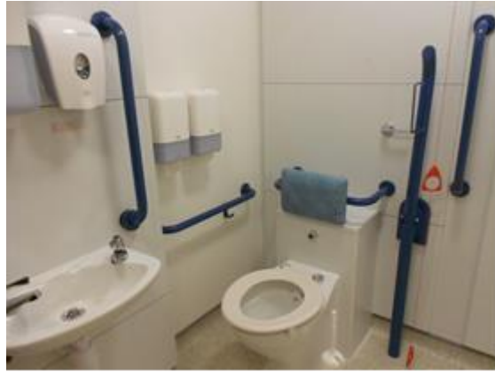
Picture 4: An example of a clean and tidy toilet with hand and grab rails and emergency pull cord
