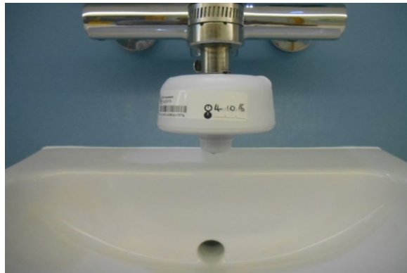
Picture 2: Point of use filter with missing removal date
