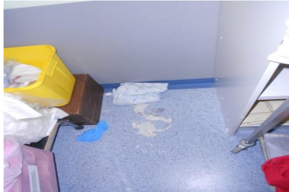
Picture 2: Debris on the floor of the linen store
