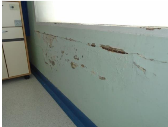
Picture 3: Damage to the paintwork and plaster around window frames in patient bay
