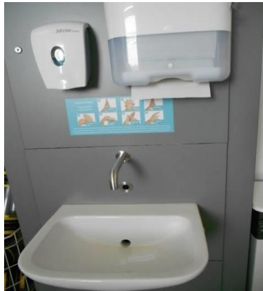
Picture 5: Ingrained dirt at IPS panel joint above hand wash tap
