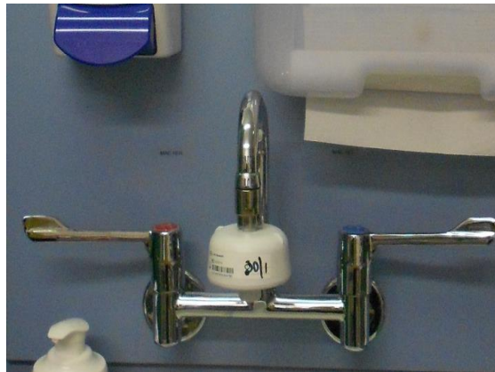
Picture 2: Point of Use filter with no removal date
