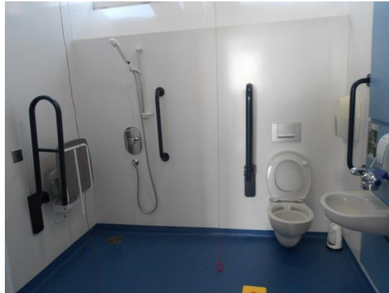
Picture 7: Refurbished shower room
