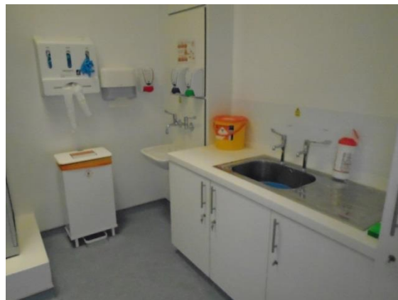
Picture 1: New equipment Decontamination Room
