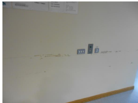
Photo 2 Recent damage to wall caused by mobile patient equipment
