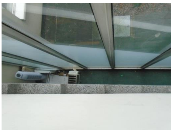
Picture 1: Area under the stairwell with visible build-up of dust, debris and clutter
