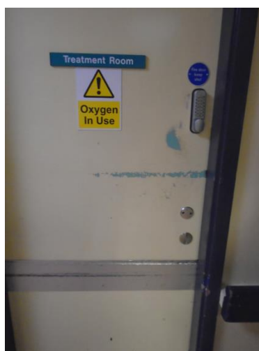
Picture: 3: Damaged paintwork treatment room door.
