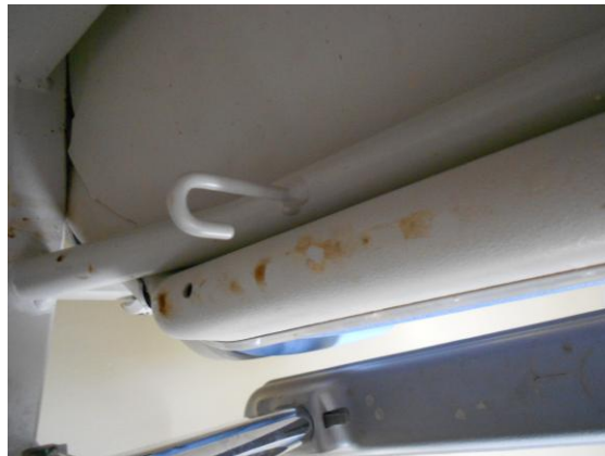
Picture 2: Stained underside of chair in day room
