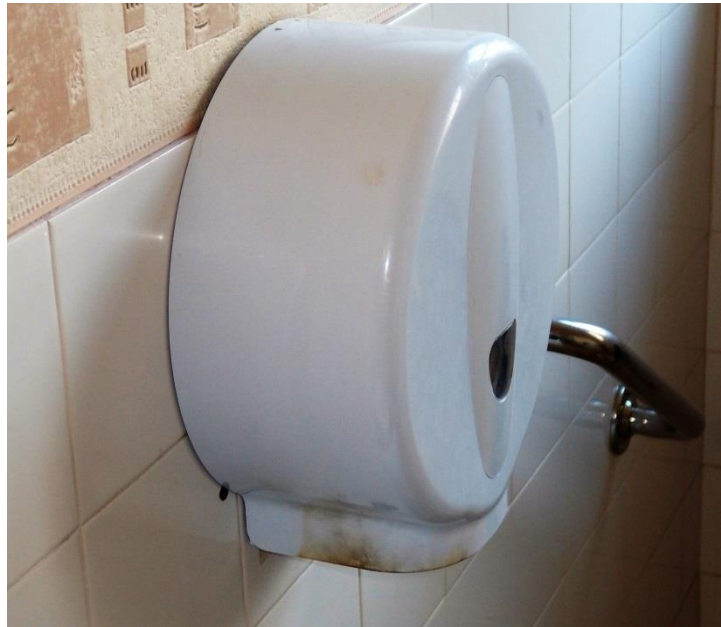
Scorch Damage to toilet roll dispenser in first floor bathroom
