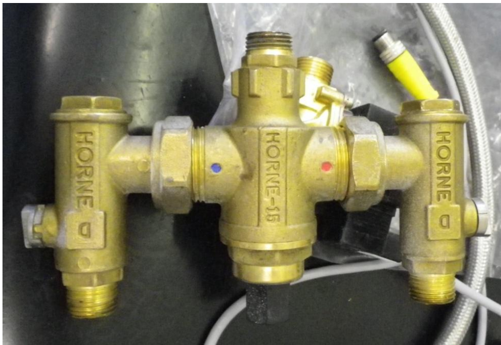
Figure 2.2. Solenoid and thermal mixing valve from Ulster Hospital, Dundonald.
