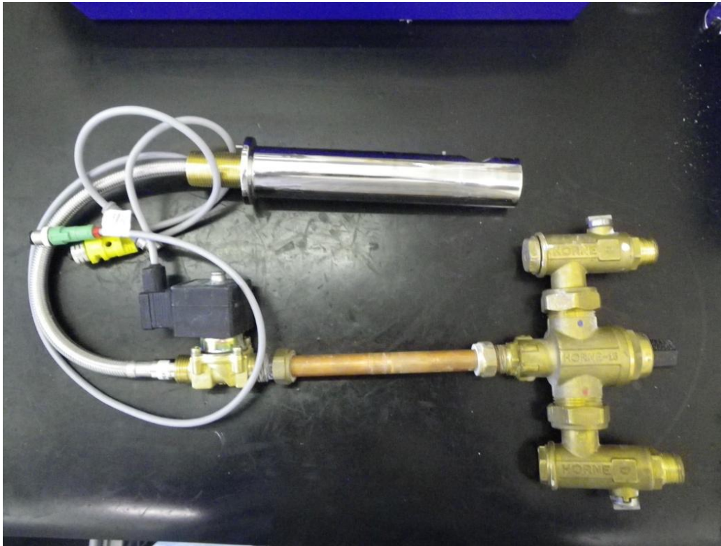
Figure 2.1. Tap assembly and components with flexible hoses from Ulster Hospital, Dundonald.
